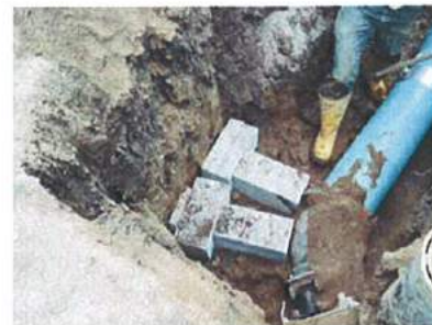
PVC pipe has a thinner wall and is lighter than comparable materials, yet still has an HDB of 7,100 psi.
