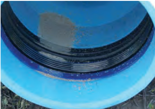
Figure 1: The sand and grit shown above must be cleaned from the restraint hardware. Dirty hardware may prevent the restraint mechanism from working.
