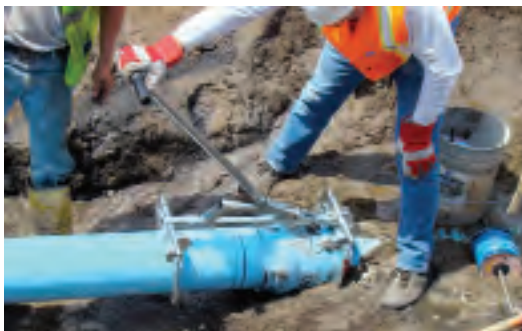
Figure 11: This assembly tool is called the Eagle Claw and is available from Pro Pipe Solutions.
