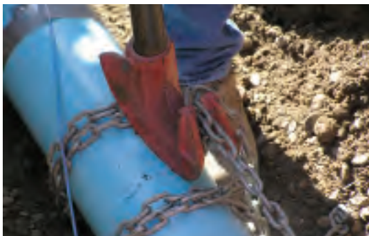
Figure 12: This assembly tool uses a chain wrapped around the bell and a lever bar to make the joint.
