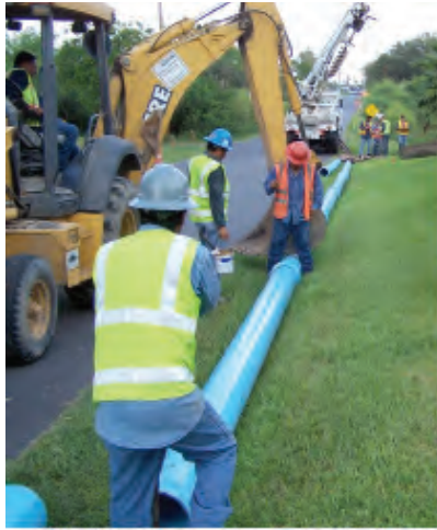
Figure 7: Example of an Eagle Loc joint assembly
